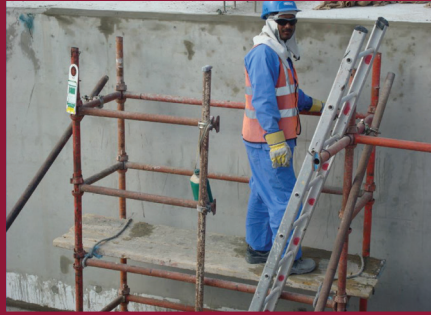
COMPLETE SCAFFOLD WORKING PLATFORM WITH INSPECTION TAG
