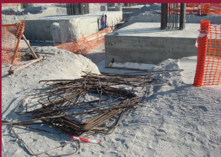
IMPROPER STACKING OF MATERIALS POSES TRIPPING HAZARD
