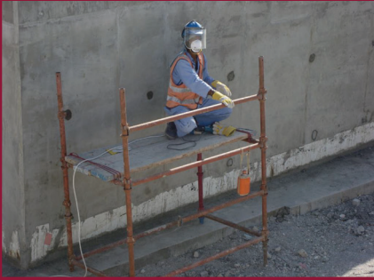
INCOMPLETE SCAFFOLD PLATFORM USED WITHOUT INSPECTION TAG
